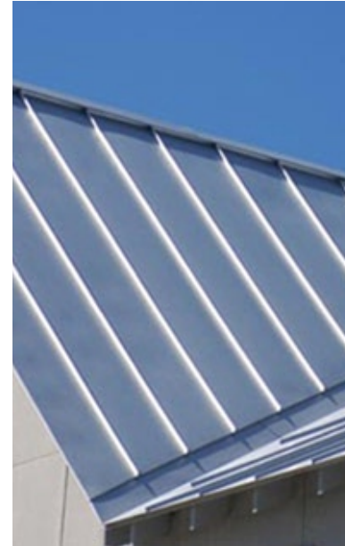
Standing Seam Metal Roof
