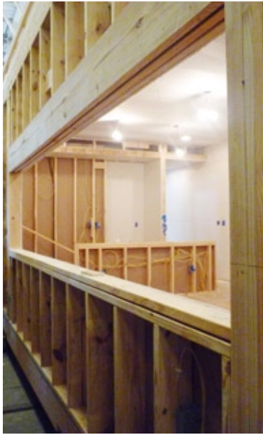
2 x 6 Exterior Wall Construction
